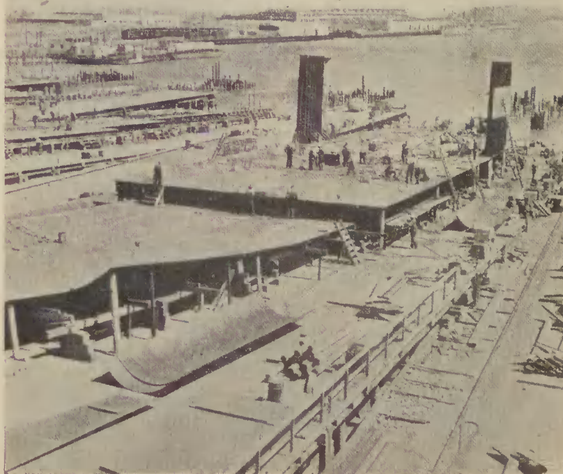
First section of double bottom and side framing erection.
