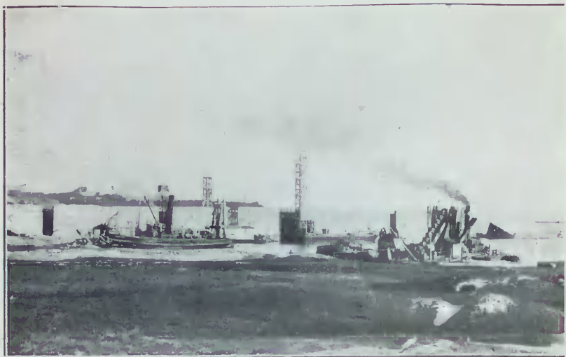
Dredging of the inner canal and caissons.
