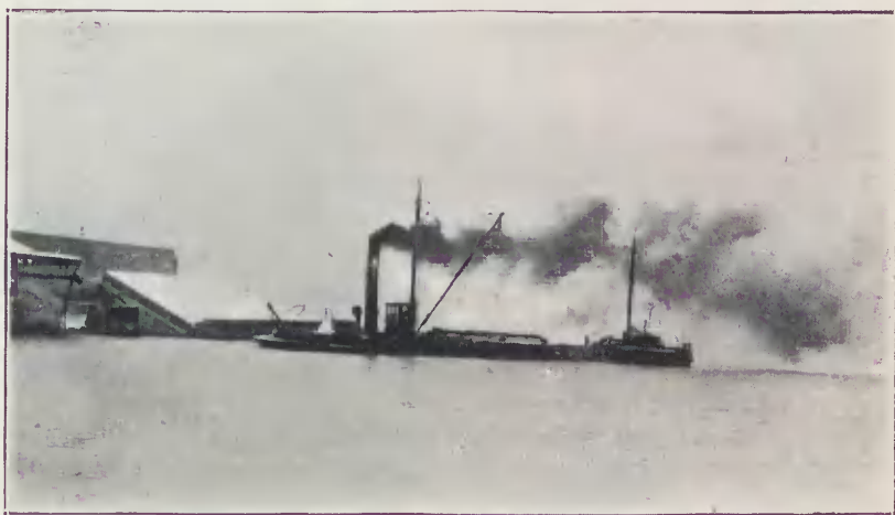
Suction-dredge and caisson in the process of floating.
