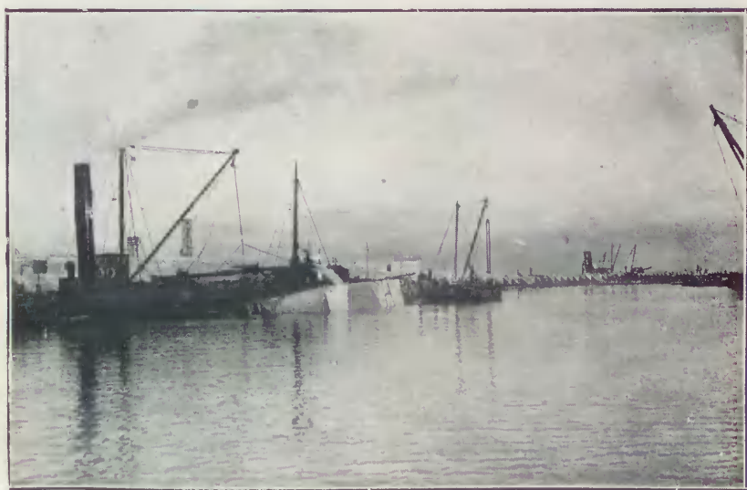
Ferro-concrete caisson half-aflloat.
