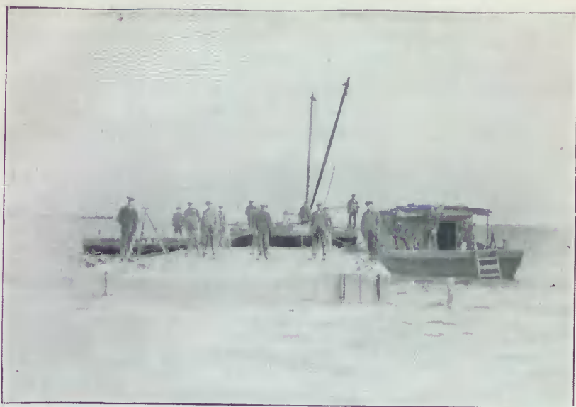
Sinking of a ferro-concrete caisson in its exact final location.
