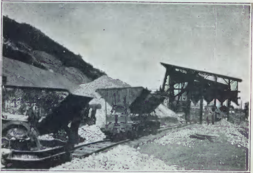
Unloading of rock boulders and road metal for port construction.
